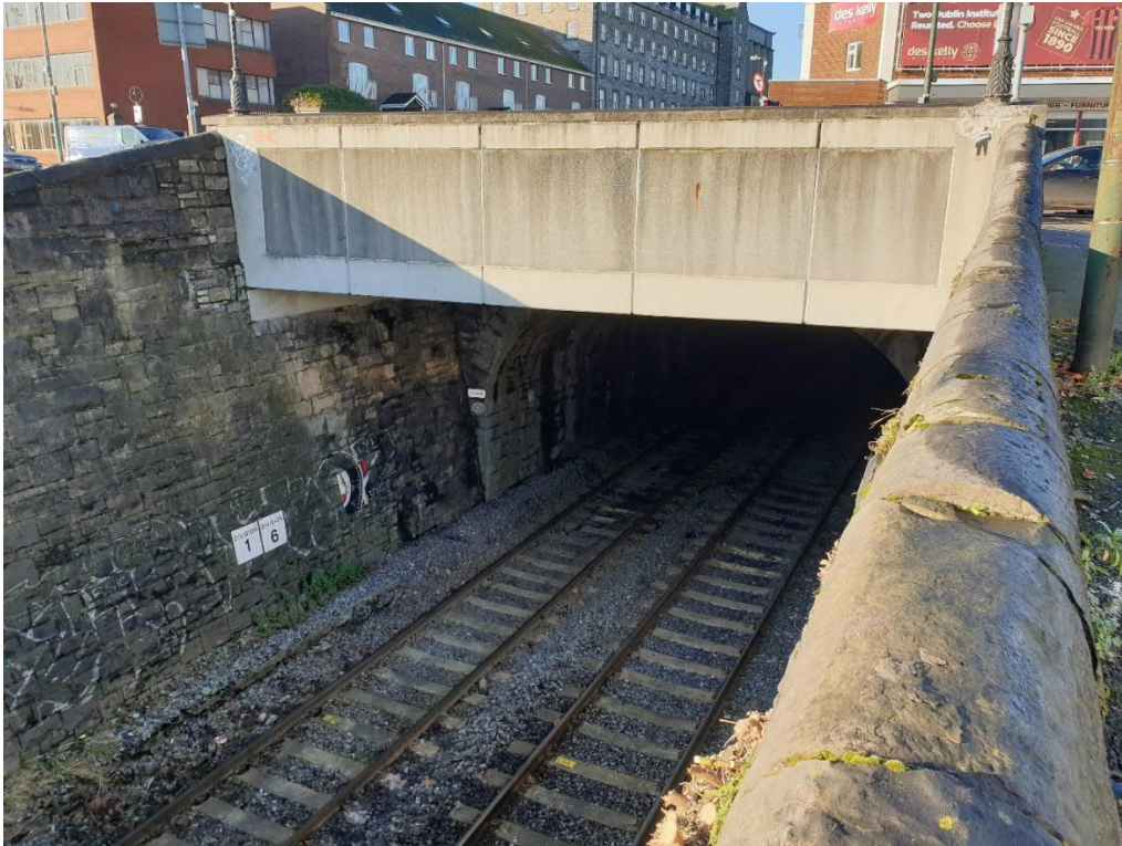
View of railway tracks – location of proposed Ballymun 02
