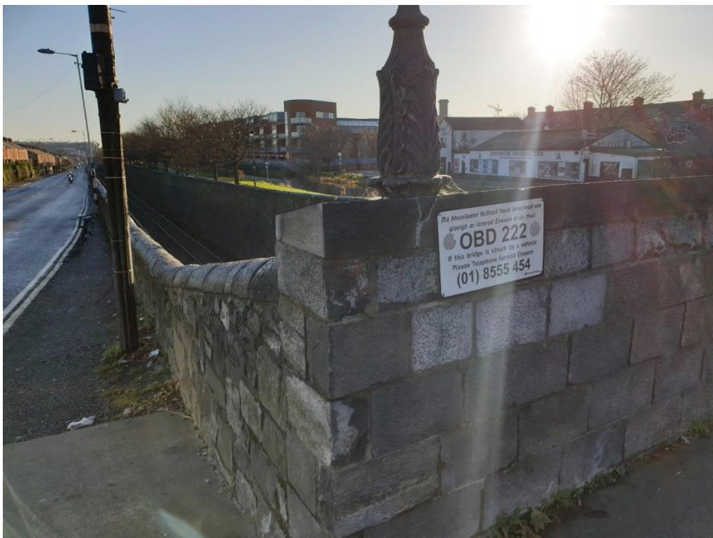
Existing parapet to be partially demolished
