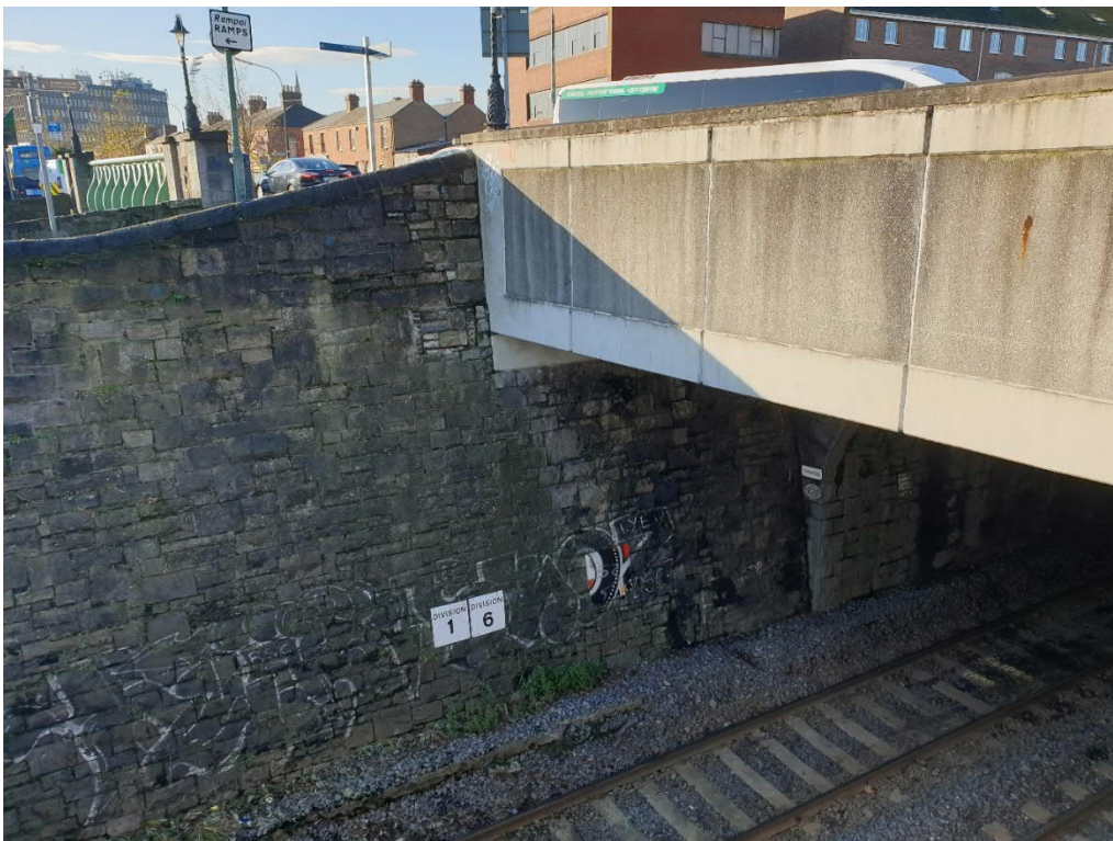
Existing retaining wall at the location of proposed Ballymun 02
